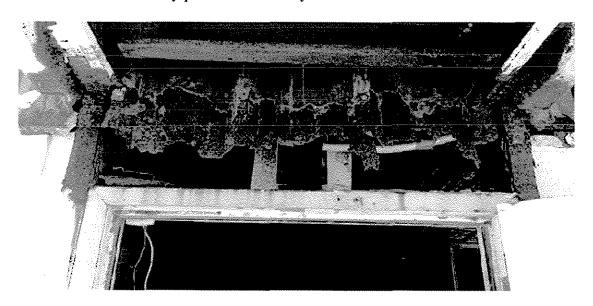
According to some advisors and professionals in the field of insulation, health hazards from this specific insulation can be actually absorbed through the skin of people using the gym, additionally, the insulation is also considered obsolete and should not be used when constructing.
